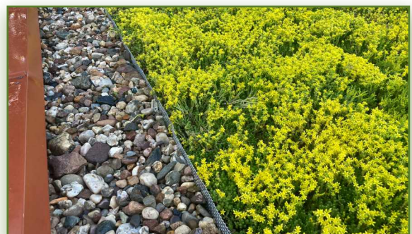
7. Place the rolled up vegetation blanket carefully on the substrate with the blanket flap downward. Unroll carefully. Put crumbled off vegetation back in place. Use the knives to cut the mats around roof penetrations. Use left-over pieces / plant chunks to fill in bare spots. Water immediately after, the installation.
