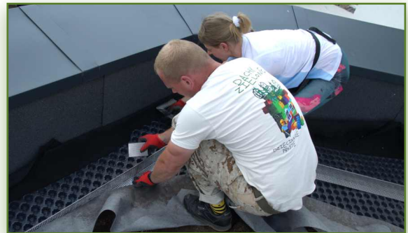
4. Make a gravel strip using separation profiles Greenfond LS-P
