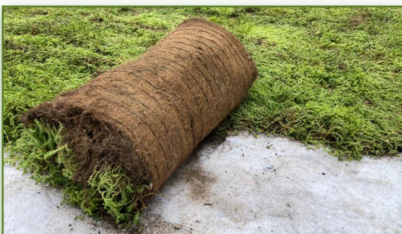
7. Place the rolled up vegetation blanket carefully on the substrate with the blanket flap downward. Unroll carefully. Put crumbled off vegetation back in place. Use the knives to cut the mats around roof penetrations. Use left-over pieces / plant chunks to fill in bare spots. Water immediately after, the installation.
