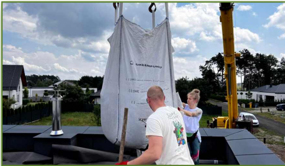
1. Prepare the ground for the mats.
