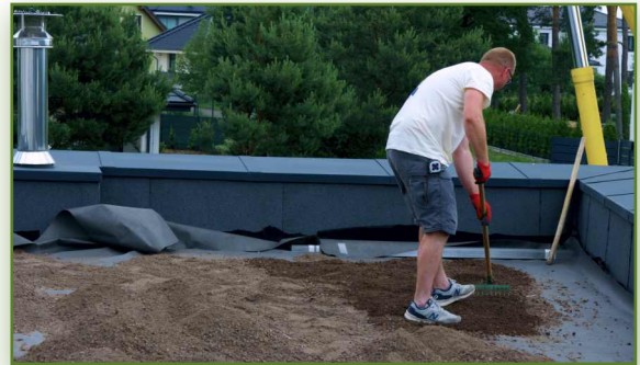
2. Level the substrate
