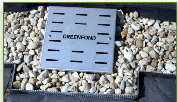
6. Place the Greenfond SK inspection chamber over the water inlet
